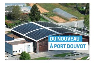
The Besançon wastewater treatment plant, which treats wastewater from Besançon and 28 other municipalities with a total population of around 150 000, has had a positive energy consumption balance since 2022. It is due to the production of photovoltaic electricity, which is immediately consumed by the site's installations, to geothermal energy, which is also consumed on site, and above all to the production of biomethane from its methanisation, which is fully injected into the GRDF network.
