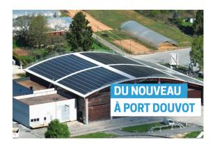
The Besançon wastewater treatment plant, which treats wastewater from the city and 28 other municipalities with a total population of around 150 000, has had a positive energy consumption balance since 2022. It is due to the production of photovoltaic electricity, which is immediately consumed by the site's installations, to geothermal energy, which is also consumed on site, and, above all, to the production of biomethane from its methanisation, which is fully injected into the GRDF network.
